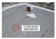
During a 2021 roof inspection the inspector's foot broke through the rubber roof and underlying rotted roof boards.
