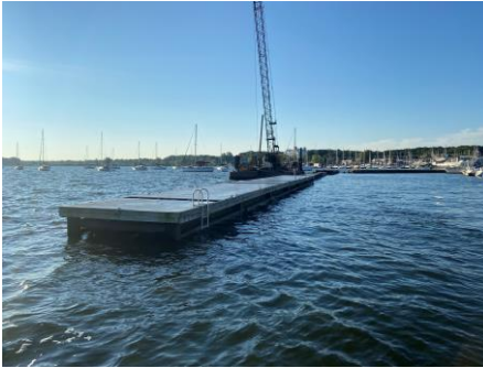
The final alignment of the outer wave attenuator
