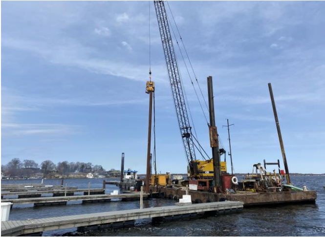
Driving new piling to provide additional support to "B" dock.
