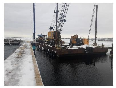
is lifted by the crest of a wave and the other sections are down in the trough of the wave. This constant twisting and torquing action have snapped 18" wide I-beams in half. The fix is to have the sections separated 12' to 15' and have bumpers in between them and let them rock & roll on their own. This will defuse the waves from doing damage to our inter marina. Unfortunately, with the sections being separated, you would not be able to walk between them.
