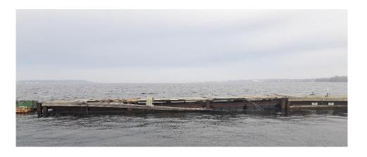
Additionally, in November we had two 13" diameter plying's (see pic) installed at the end of the finger piers of slips 5 & 6 and 8 & 9 on "A"
