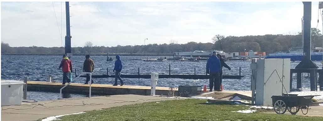
It was a cold morning installing the bubblers....brrrrrr!
