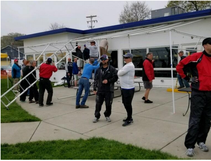
The extra 8" in height added to the awning frame made for a difficult install. Melges 24 sailors jumped in and lent a hand.
