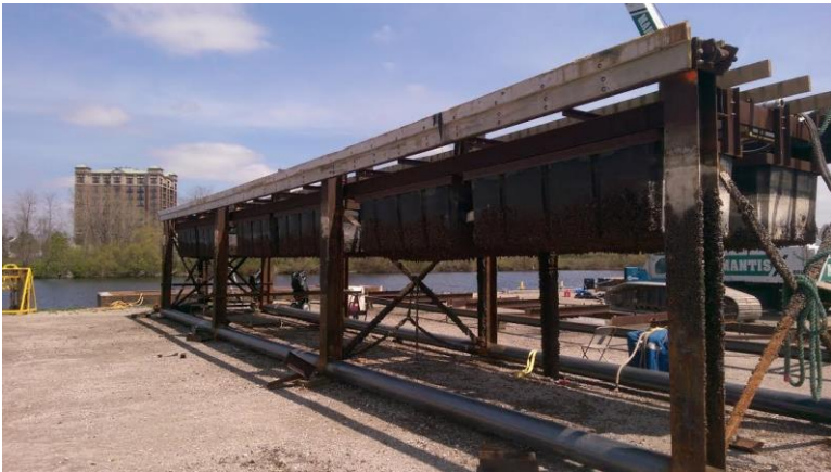
Four dock sections rebuilt. A fifth section is already back in the water.
